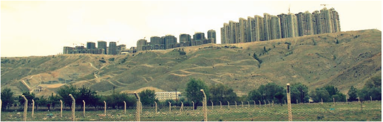
Figure 13. The Photograph of the housing project from the İmrahor valley basin (Source: the author, 2014).
