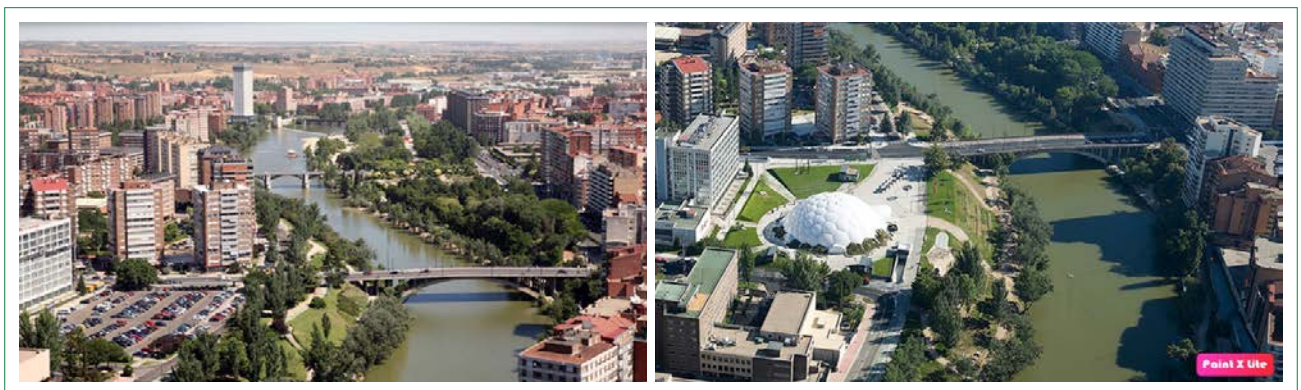
Figure 2. Millennium Square project area before (2009)/after (2011) implementation (Ruiz-Geli, 2012, Photos by Luis la Forga and Tafyr respectively).
