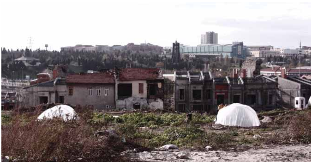
Figure 1. New construction taking place in the old neighbourhood, Sulukule. Photograph: Can Berkol, 25.11.2010.
