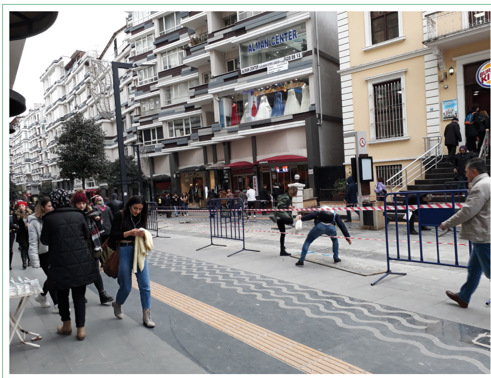
Figure 5. Preparations for reopening the traffic on Çiftlik Street (Photo by author).
