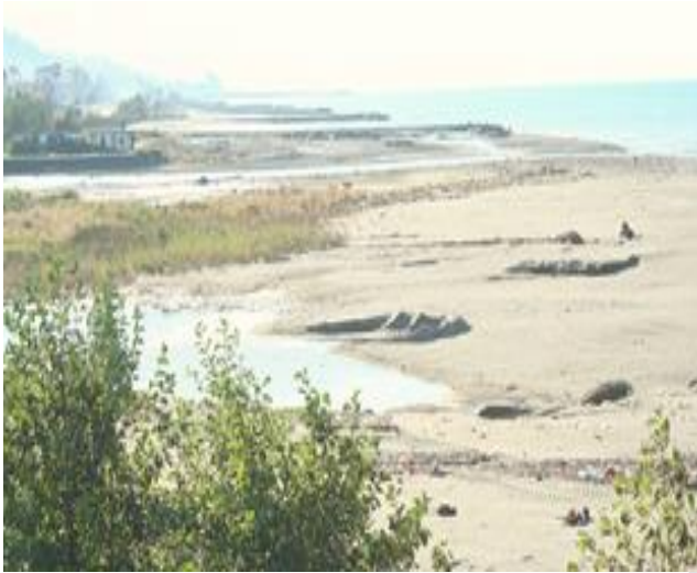
Figure 17. The effect of the flood on T-shaped groins
