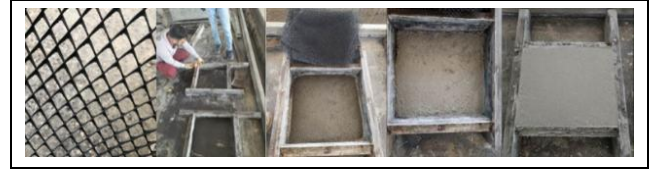
Figure 4. Concrete formwork with geogrid and pouring.
