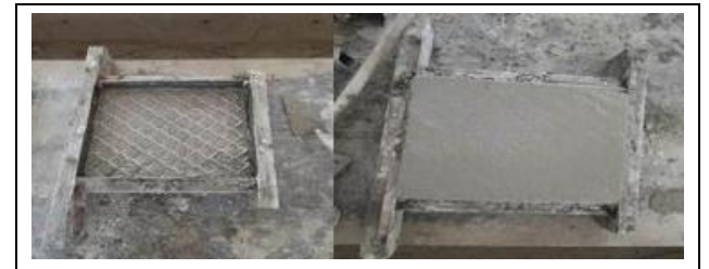
Figure 6. Concrete formworks of prepared Galvanized Wire and pouring.
