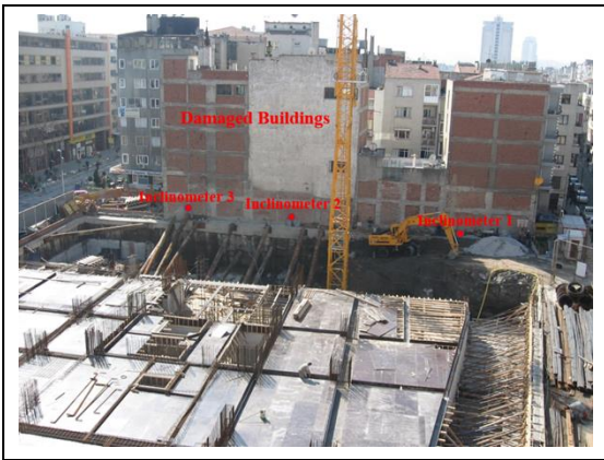
Figure 5. View of the subject building and the location of the inclinometers.
