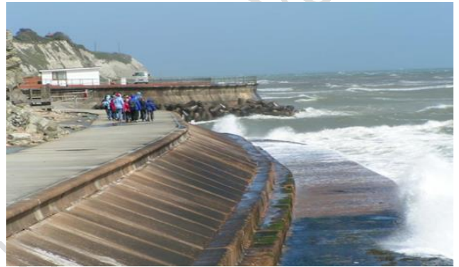
Figure 8: An example of a modern seawall on England's Isle of Wight [93].
