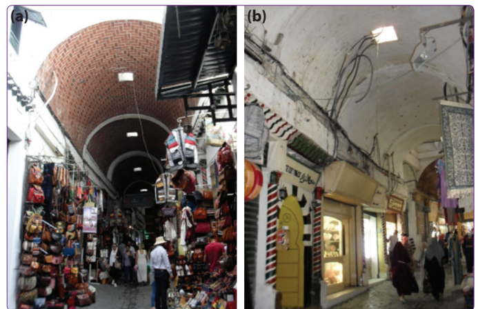
Figure 8. (a) Entrance of "Al-Truk" bazaar, (b) Electricity and air cooling cables in the bazaar's roofs (Provided by 1 st author taken on 20 th of July 2016).
