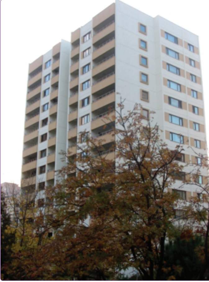
Figure 5. Feneryolu Apartment (1958-1967) in Kadıköy/Istanbul (Eren, 2014).
