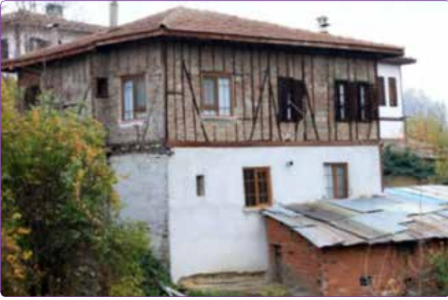
Figure 6. Additional structure adjacent to housing structure.
