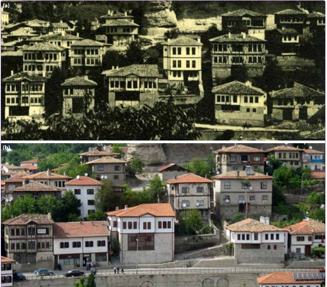
Şekil 8. (a, b) Two Photos of the Same Area (Figure 8a: The photo, date unknown taken from the Safranbolu Municipality Archives, indicates a plethora of plastered buildings that leave the unplastered/wooden frame bare. In comparison, the contemporary photo reveals the increased tendency of covering these wooden frames with plaster.)
