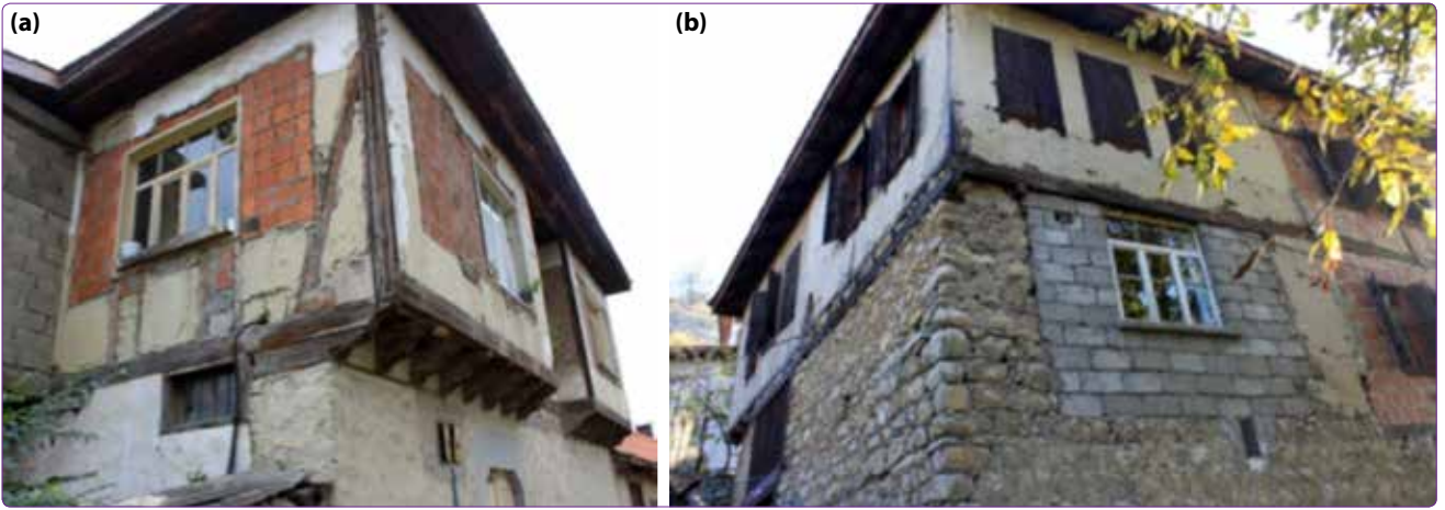
Figure 9. (a, b) Renewed windows.
