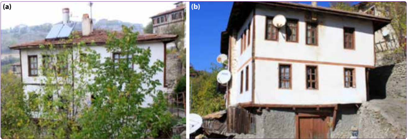
Figure 10. (a, b) View of solar energy panels and dish antennas.
