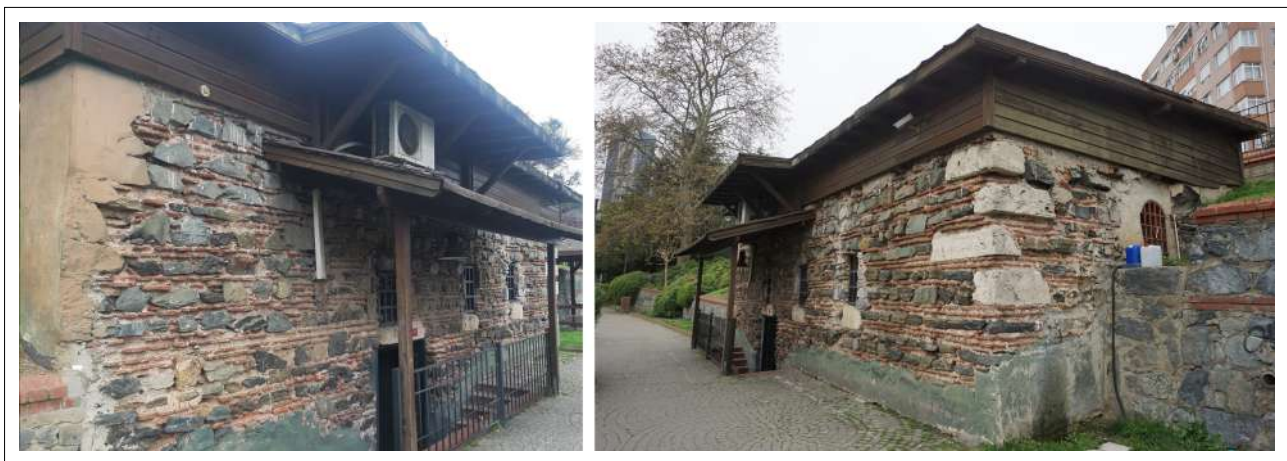
Figure 14. The existing structure of B4.
