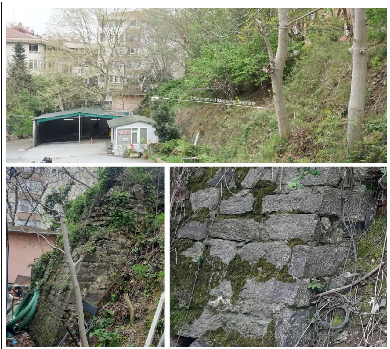
Figure 9. The embankment wall detected during the exploratory field survey.
