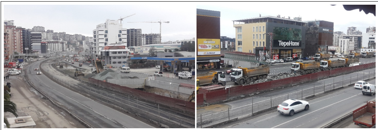
Figure 4. Construction activities of Kaşüstü junction project (Fieldwork photos of November 2018).
