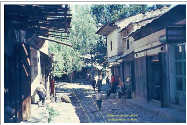
Figure 6. Water ditch that allows surface water to flow in historic streets of Beypazarı (Source: Beypazarı Municipality).
