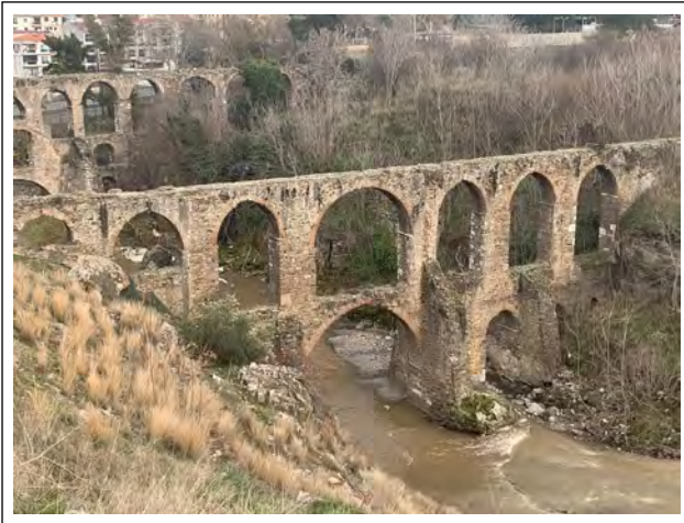
Figure 2. Akvadük Aqueducts in İzmir, Turkey (Eken Güney, 2020).
