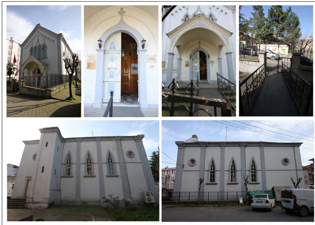
Figure 1. Outdoor structural elements of Giresun central children's library.
