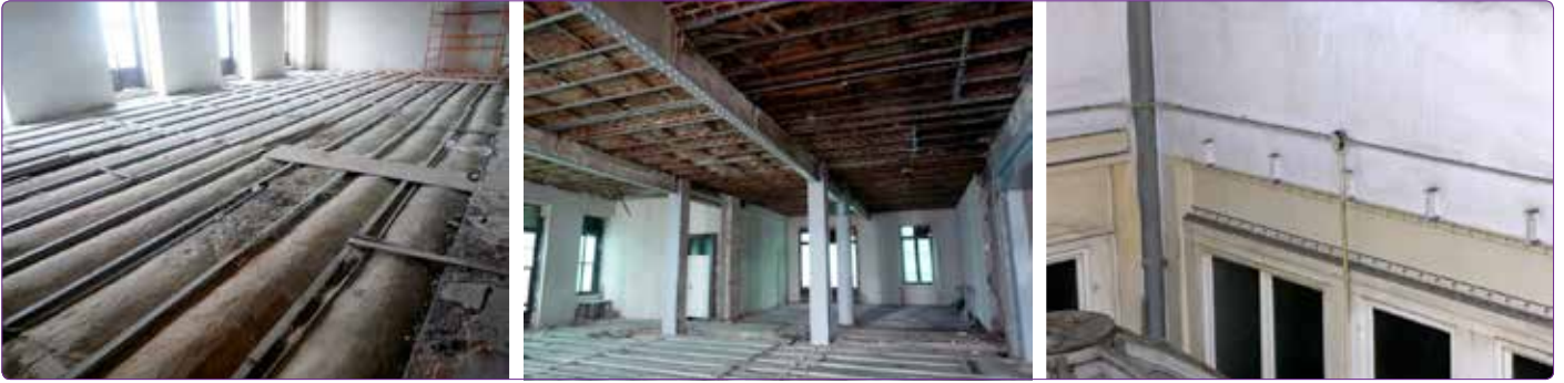
Figure 6. Arched floor system of Pera Palace Hotel.
