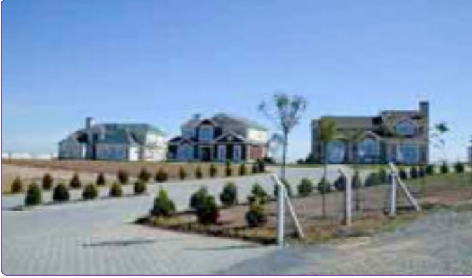
Figure 3. Tepe Ören Villas.
