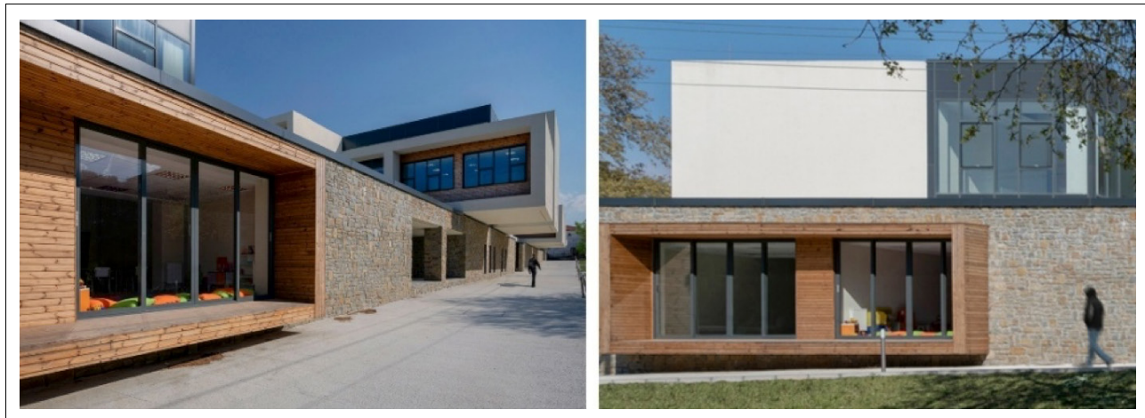
Figure 16. The facade of the workshops on the İnönü Street side (Arkitera, 2019).
