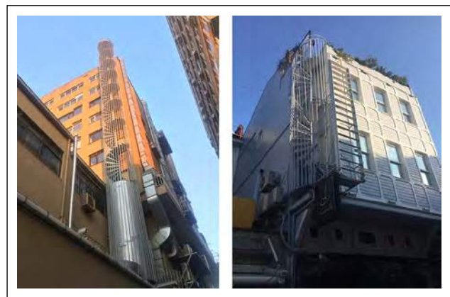
Figure 13. Hazard sources Nos. 10 and 14.
