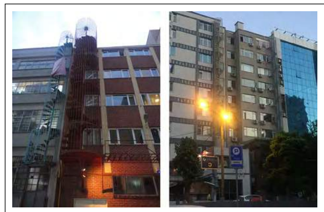
Figure 9. Hazard sources Nos. 12 and 16.
