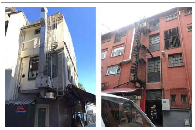
Figure 8. Hazard sources Nos. 1 and 2.
