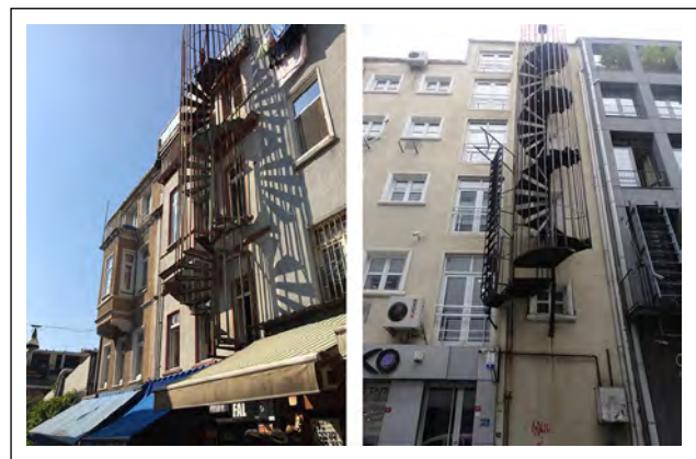
Figure 11. Hazard sources Nos. 8 and 9.
