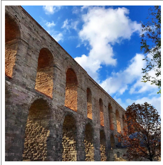
Figure 2. Bozdoğan (Valens) Aqueduct.
