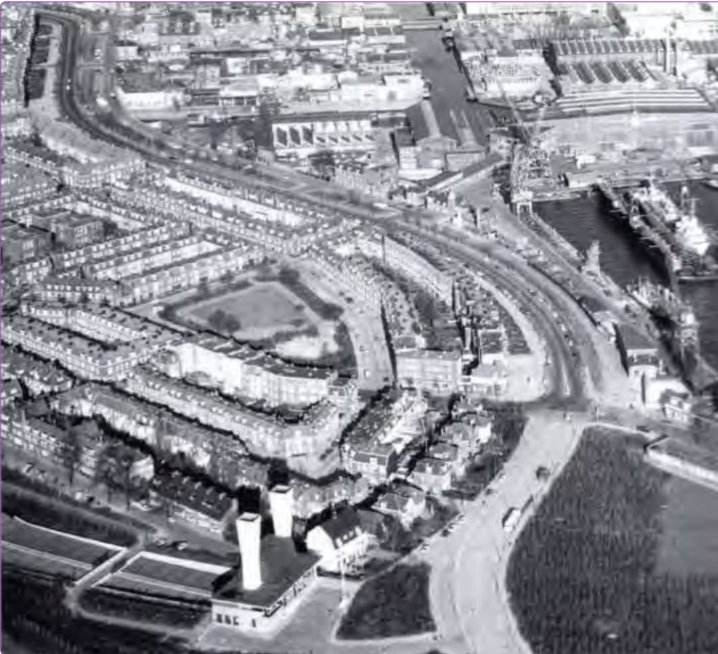
Figure 6. Vogelbuurt area before construction of housing on the IJ-plein, 1970s (Source : Jolles, A. (2003) Planning Amsterdam: scenarios for urban development, 1928-2003, Rotterdam, NAI Publishers, p. 146).
