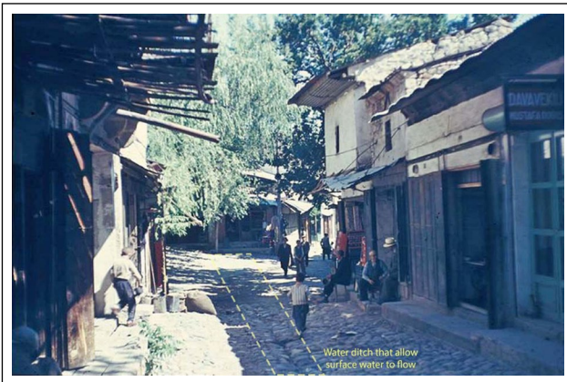
Figure 6. Water ditch that allows surface water to flow in historic streets of Beypazarı (Source: Beypazarı Municipality).
