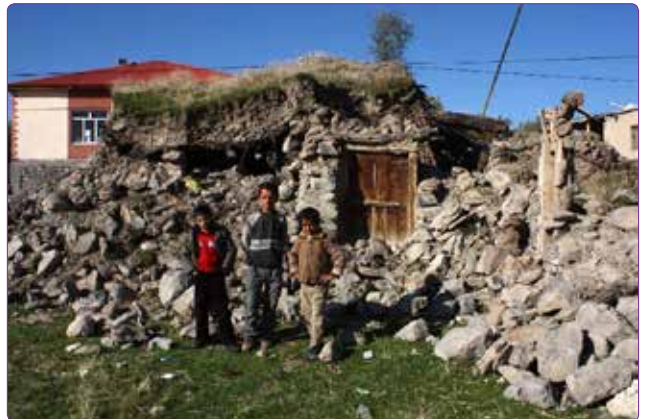
Figure 10. A heavily damaged building with mud ceiling (Parsa, A.R. Archive, 2011).
