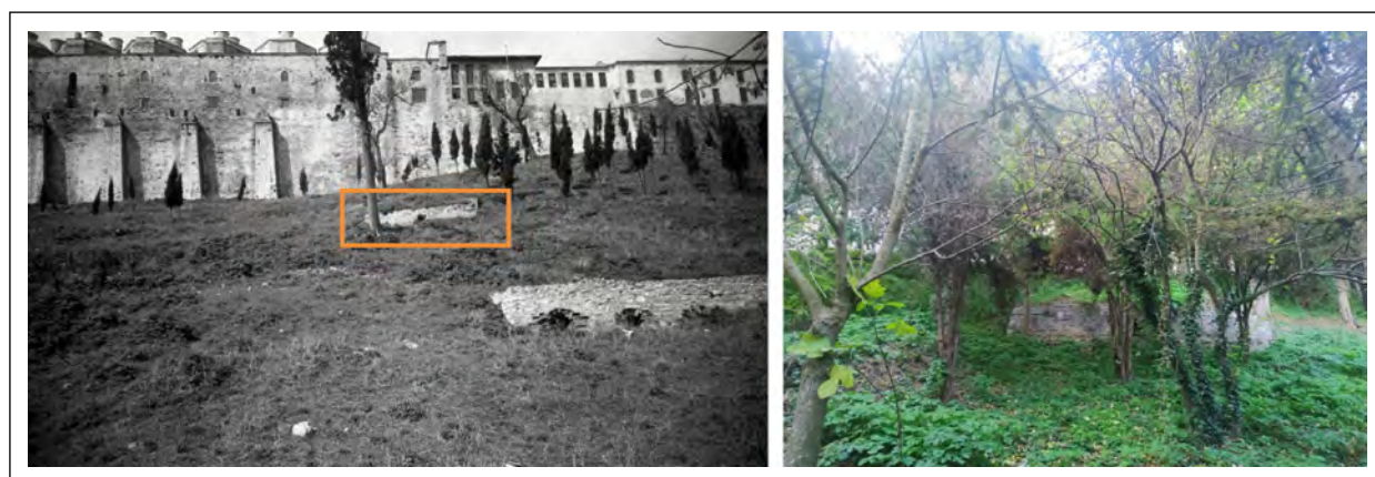
Figure 16. The remain assumed as a water tank is located at the palace garden behind the kitchens. The photo on the left was taken by Ayverdi in 1940’s (EHAEA, 1940-1944). The photo on the right shows its current condition (Uysal Eng dar, 2021).
