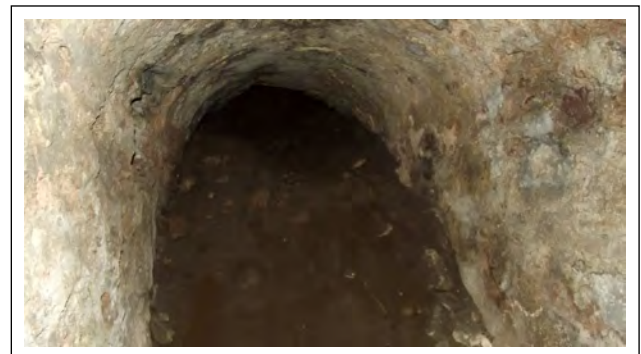
Figure 8. Vaulted drainage underground channel at the kitchen court (Özbersan İnşaat ve Ticaret Ltd. Şti., 2013).
