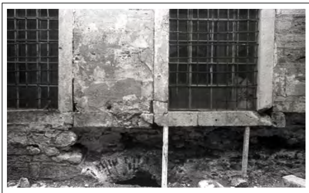
Figure 18. The brick arch on the kitchen’s wall during restoration between 1940 and 1944 (EHAEA, 1940-1944).
