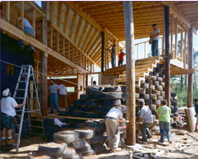
Şekil 2. Rural Studio 2002, Shiles House Uygulama (URL-1: http://www.ruralstudio.org/projects ).
