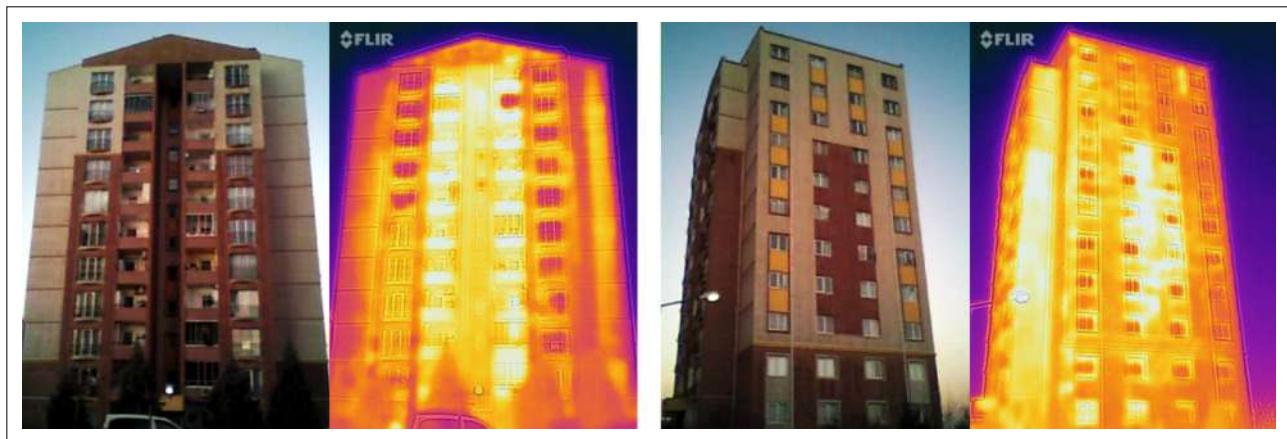
Figure 11. Exterior wall temperature on the southwest (left) and southeast (right) façades of Block 3 in TOKI Etiler in December (Photo by Bay-Şahin, 2019).
