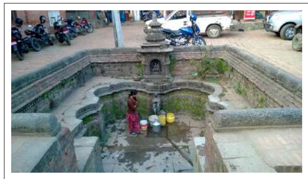
Figure 11. The traditional water supply system in the Kathmandu Valley is utilized for both daily needs and emergencies (Jigyasu, 2015).
