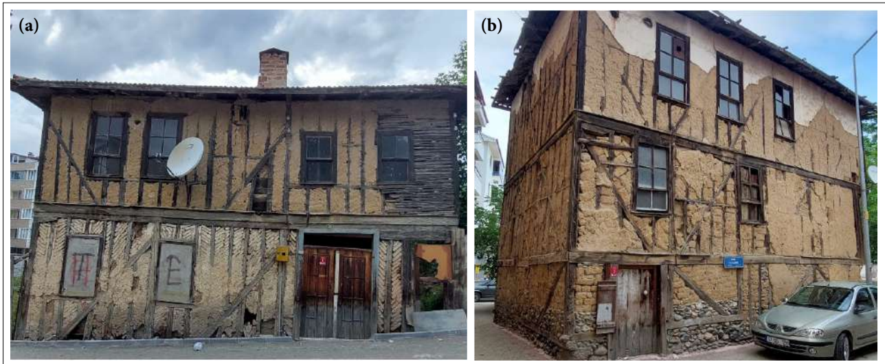
Figure 3. (a) Example of Hımiş and partial bağdadi structure, (b) Basic stone filling hımiş system structure.
