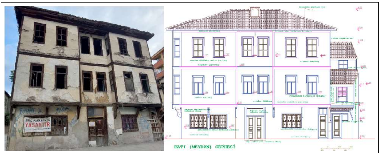
Figure 9. West facade of Mehmet Kaya House.
