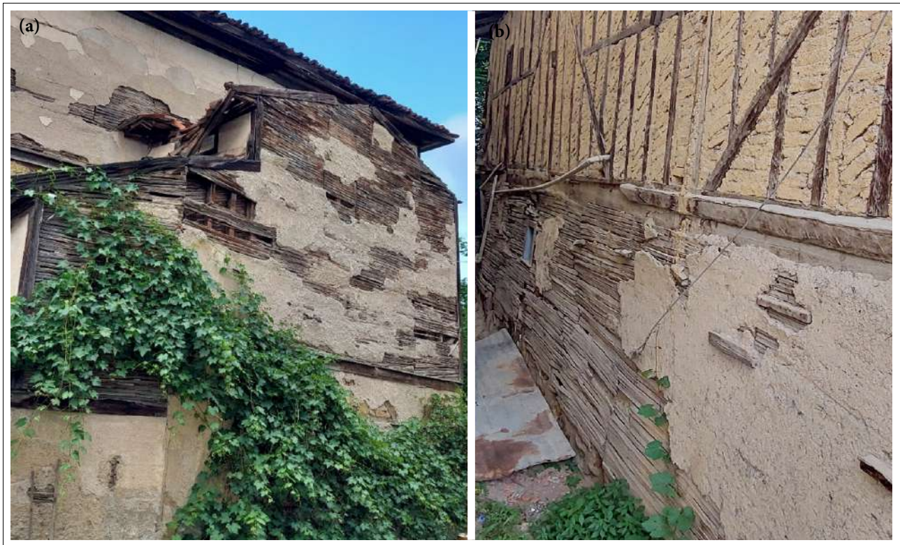
Figure 2. (a) Bağdadi system technique (Sinop) (b) Bağdadi and half-timbered system technique (Sinop).
