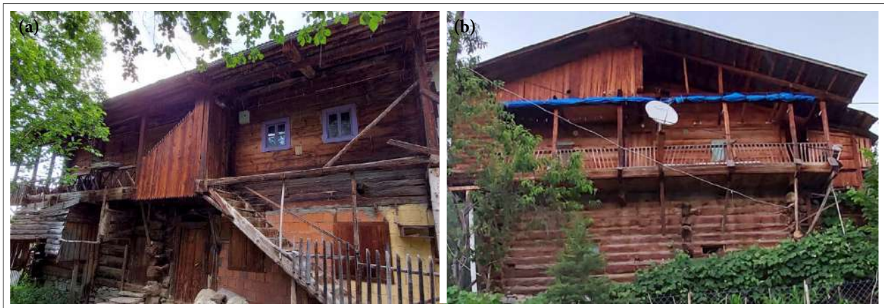
Figure 1. (a, b) Examples of timber structural systems created by sequential alignment of planks and logs Artvin/Türkiye.
