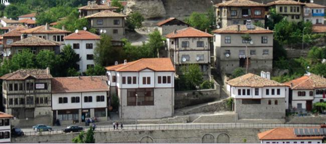
**Şekil 8. (a, b)** Two Photos of the Same Area (Figure 8a: The photo, date unknown taken from the Safranbolu Municipality Archives, indicates a plethora of plastered buildings that leave the unplastered/wooden frame bare. In comparison, the contemporary photo reveals the increased tendency of covering these wooden frames with plaster.)
