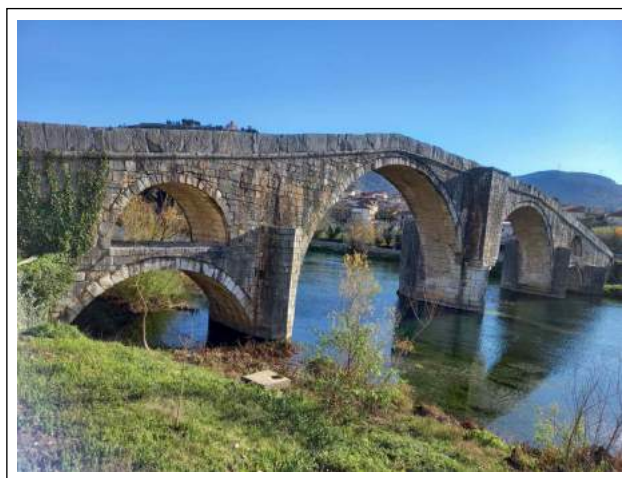
Figure 1. Arslanagić bridge in Trebinje, western facade (the photo was taken by the authors in 2022).
