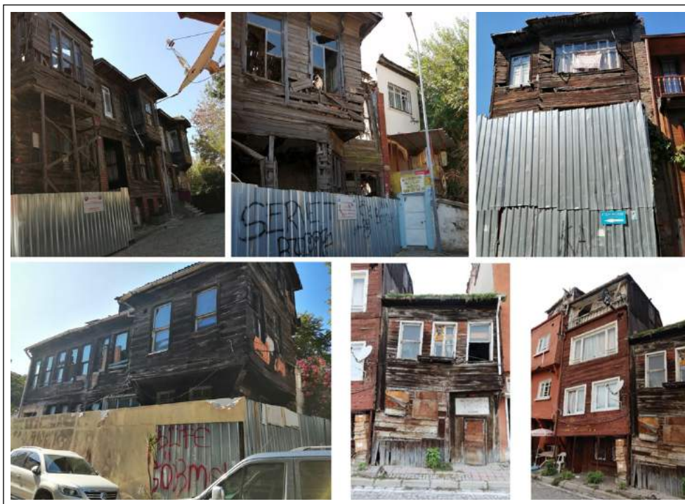
Figure 8. Deteriorations in the housing stock in the study area.
