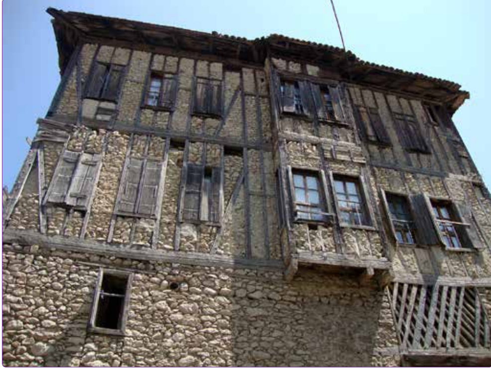
Figure 1. A traditional timber framed building with stone infill in Safranbolu.
