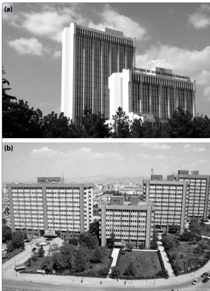
Figure 4. The Ministry of Employment and Social Security (a) and the Ministry of Culture and Tourism (b) constructed until 2000s (Source: Author's archive, 2017 (a) and Emek Construction, 2020 (b)).
