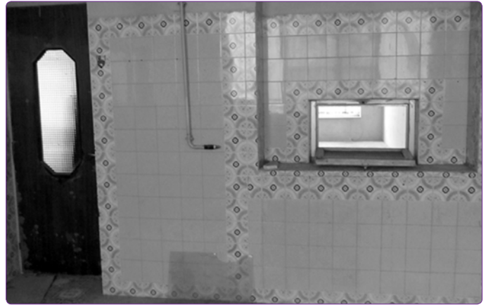
Figure 16. The connection of kitchen to the dining area through a small fenestration.
