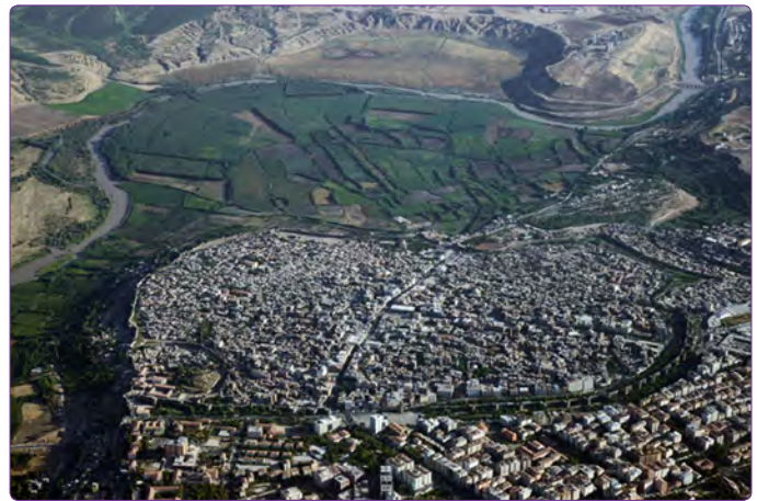
Figure 8. City walls, Hevsel Gardens and Tigris River (Yüksel, 2016).
