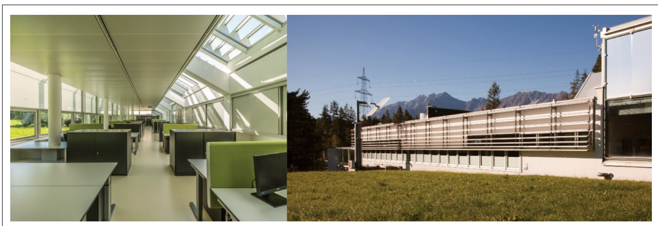
Figure 1. Interior (left) and exterior view (right) of the Bartenbach R&D building in Aldrans, Austria. In the right part of the interior area, the skylights of the north facade can be seen, the exterior view shows the static daylight system on the south facade.
