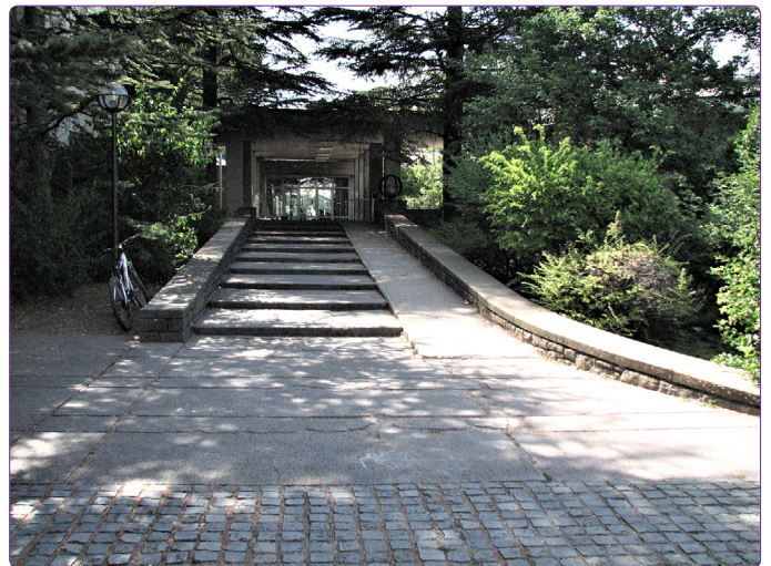
Figure 3. Inclusive access towards the Physics Building from Alley.
