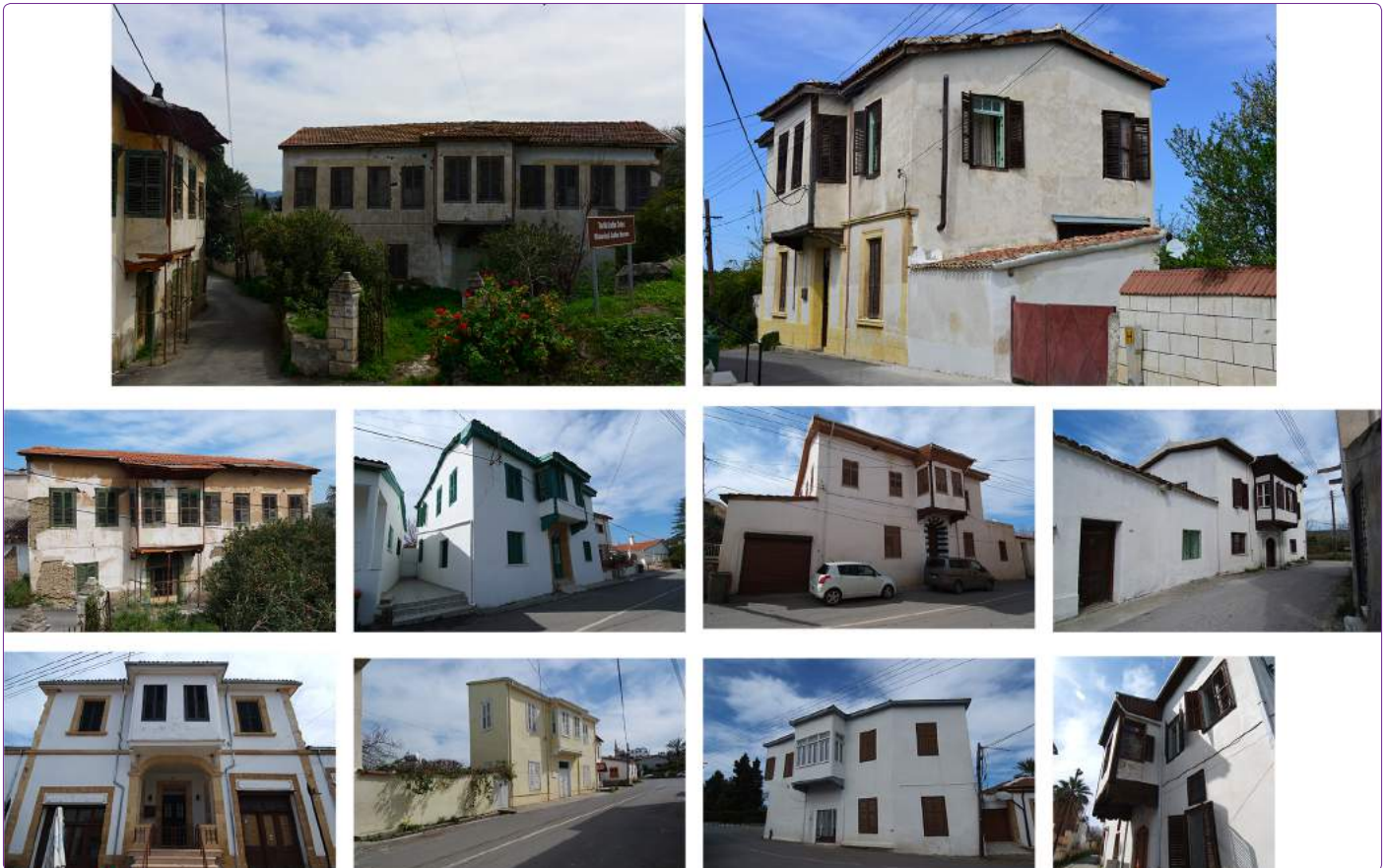
Figure 8. Two-storey traditional Ottoman houses with projecting bay in Lefke. Source: Makbule Oktay, March & April 2019.
