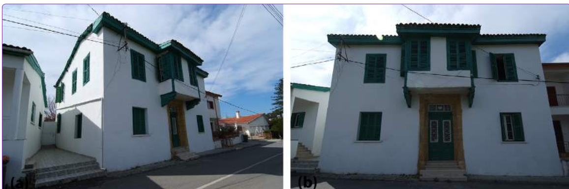
Figure 17. Sevilay Paşazade house. (a) South and east façades. (b) East façade. Source: Makbule Oktay, March 2019.
