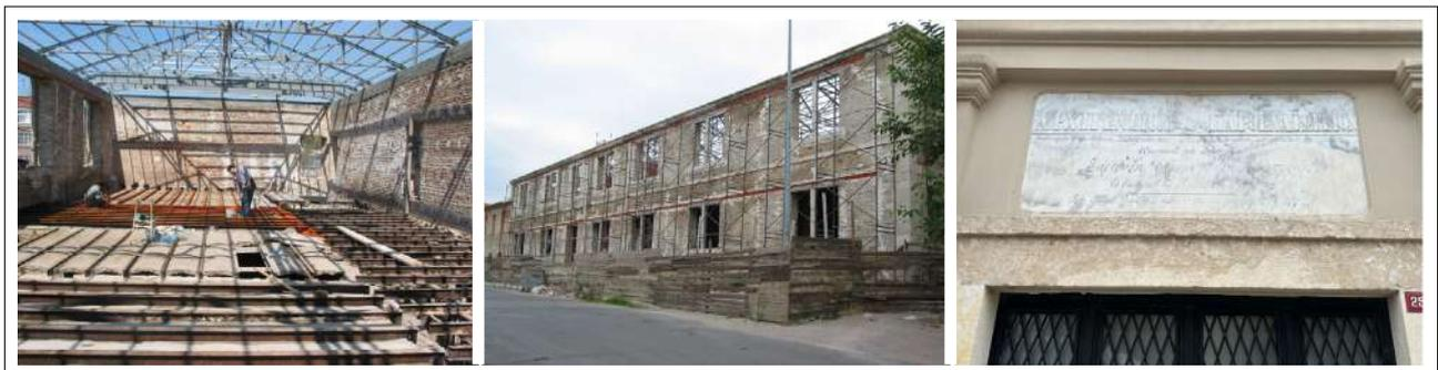
**Figure 12.** Reconstruction of the roof and floor systems during the repair of Block 2, consolidation of the brick walls, and the present state of the conserved marble inscription (Hanart Architecture Archive).
