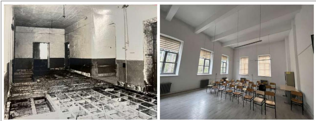
**Figure 19.** Dismantled wooden slab of the upper floor (Conservation Council Archive), Interior was reconstructed using reinforced concrete.
