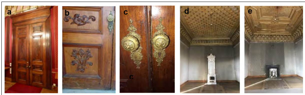
Figure 7. (a) The door made up of mahogany and walnut, (b) Mahogany rosettes on the walnut veneer panels, (c) The brass knocker instead of the silver and bronze knocker, (d) The porcelain stove of Room 105, (e) The fireplace in Room 104, 2017 (Erdem).
