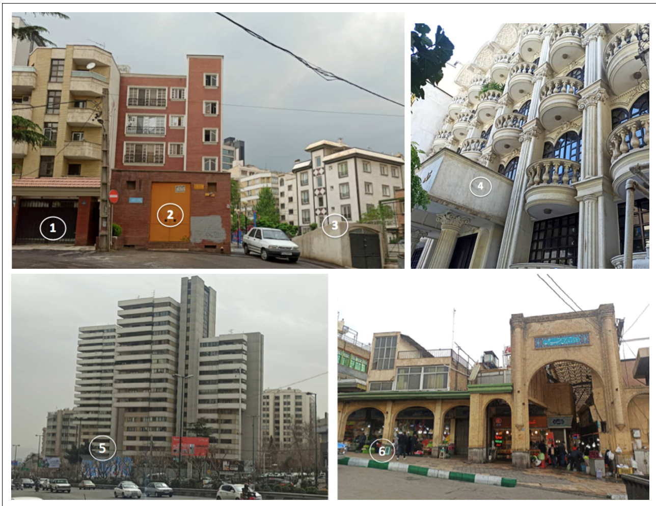
Figure 3. Facade/view, and city/ building interface of Tehran, Iran.
