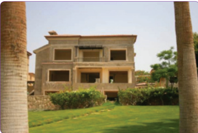
One of the interior fence models showing the diversity in creating a more private intimate space.
