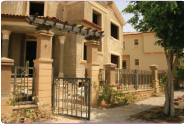
Uniformity of Villas Main Entrances.
