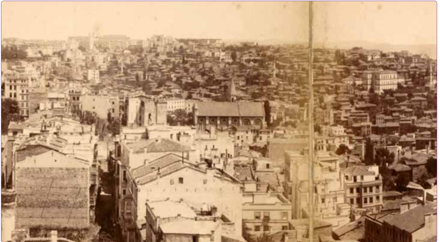
Figure 4. Masonry houses of Pera with regularized streets and the timber fabric behind, late 19 th century (SALT Research Online Archives, access code: AHISTDIV0016601E1).
