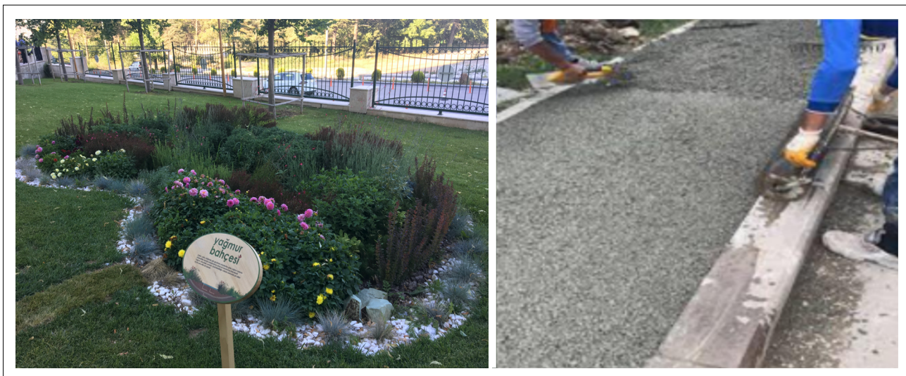
Figure 2. The implementation of permeable concrete and rain garden.
