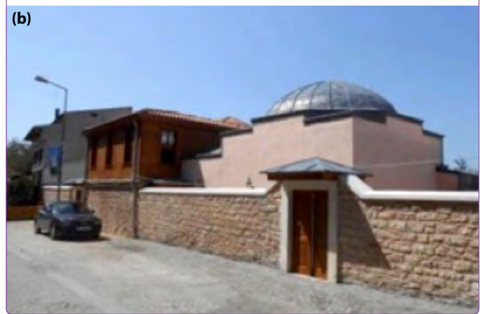
Figure 21. Merkezefedi Turkish Bath restoration; (a) Before restoration, 2007 [URL-16], (b) After restoration, 2017 (Personal archive of Authors).
