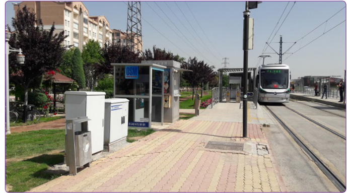
Figure 9. Bad quality pavements of Pedestrian areas providing access to tramline stations.
