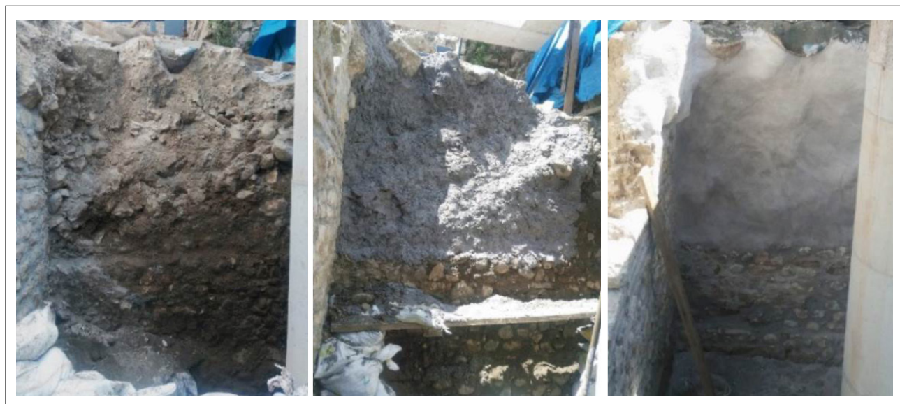
Figure 16. A weak mass consolidated by covering it with a lime mortar containing NHL 5.
