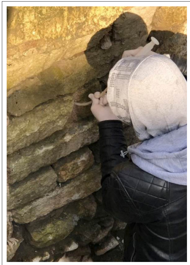
Figure 18. Grout application through injection on a wall infested with algae.
