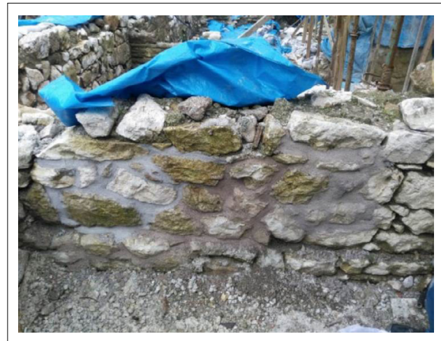
Figure 15. Previously applied lime mortar with a lighter color and fresh trial mortars with the hybrid binder (they can be distinguished by the color differences between them) applied to a small section infested by algae.
