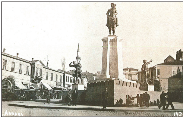
Figure 31A. Previous location of the monument, late 1920s. Source: Cangır, 2007, p. 839.
