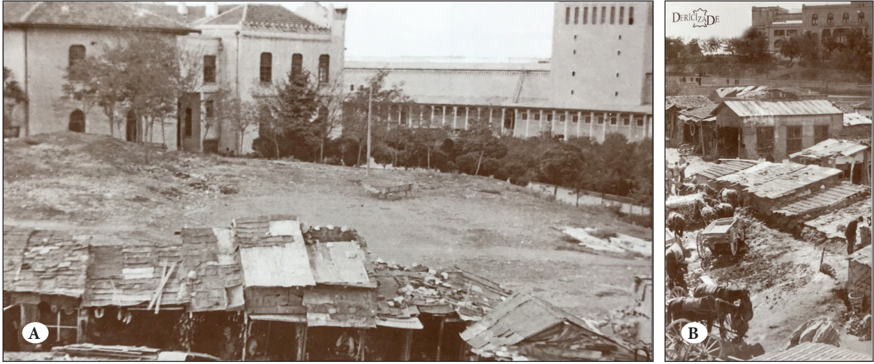
Figure 25A and 25B. Barracks erected at empty open spaces around the Ministry of Foreign Affairs.
