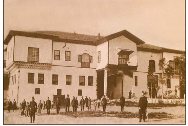
Figure 8A. The second building of Paşa Sarayı, late 19 th century.
