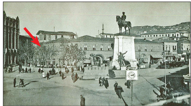
Figure 21C. Karpiç, at the entrance floor of Taşhan.
