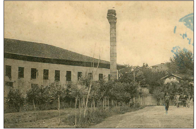
Figure 8B. Military Barrack and Julian Column in the front, 1905.
