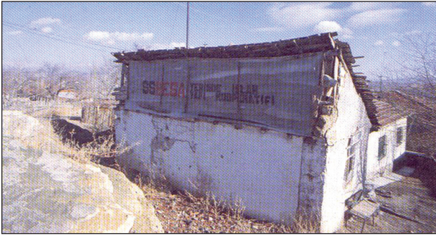
Figure 6. BESA Housing Cooperative Office. Source: Reyhan Varlı Görk's Collection, early 1990s.
