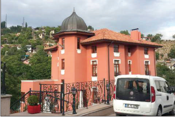
Figure 4A. İzzet Ulvi Aykurt house (Hacı Bayram Veli Quarter). Built by Hungarian craftsmen. Date: 1924-1931. Photograph by: D. Avcı Hosanlı, 2015.
