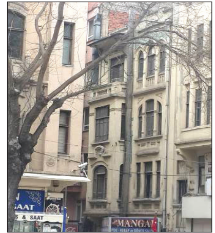
Figure 7C. Hatay Apartment (Hasan Pehlivanlı İşhanı) (Hekimler Street, No: 4). Date: before 1927.
