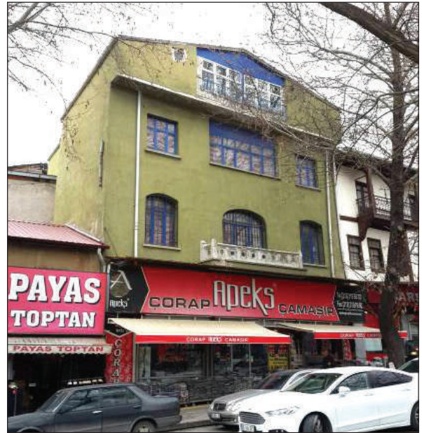
Figure 10B. A single house (Çocuk Sarayı (Anafartalar) Street, No: 89). Date: 1920s. Photograph by: D. Avcı Hosanlı, 2018.
