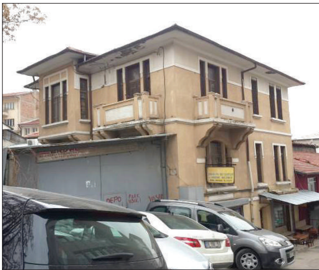
Figure 8A. A single houses (Konya-Kahraman Street, Hisarönü Quarter). Date: 1920s.
