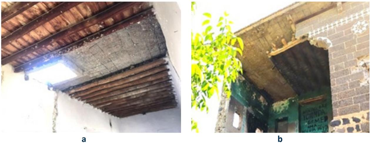
**Figure 12.** Deflection and material loss damages in wooden beams (Işık, 2021)
