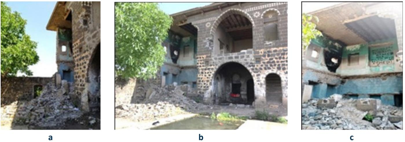
**Figure 8.** Damages on the northeastern wall of Ferit Köşk (Mansion) (Işık, 2021)
