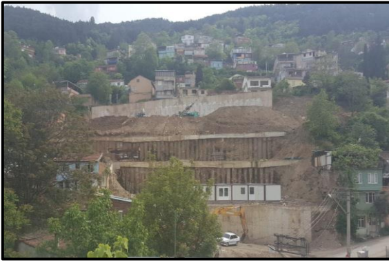
Figure 8. View of the applied support system.
