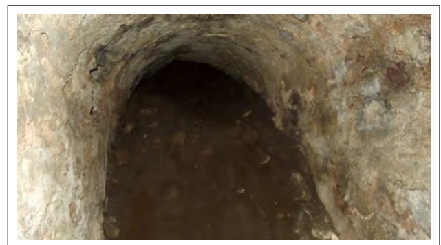
Figure 8. Vaulted drainage underground channel at the kitchen court (Özbersan İnşaat ve Ticaret Ltd. Şti., 2013).
