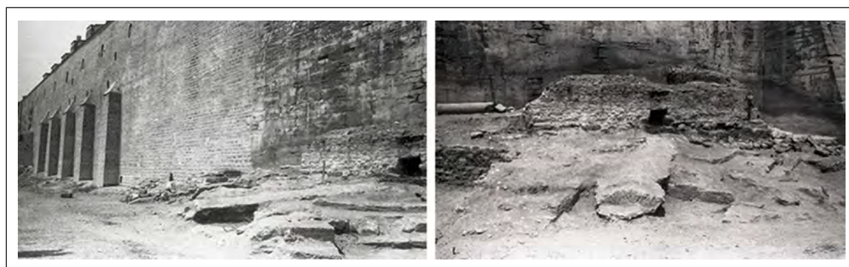
Figure 15. Left: A presumed vaulted drainage channel under the bath’s retaining wall, facing the Marmara Sea, next to the kitchens. Right: a close-up view of the channel (EHAEA, 1940-1944).
