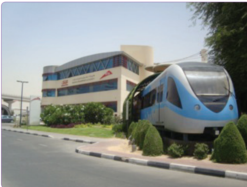
Figure 5. A representation of the Dubai Metro in front of RTA Dubai Head Office.
