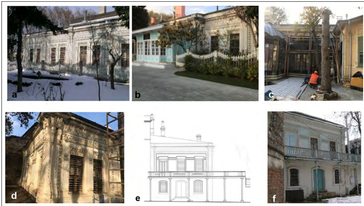
Figure 8. (a) West side of the southern facade, 2006, (b) The main entrance, southern facade, 2017, (c) Greenhouse (eastern face) 2018, (d) Southwest corner of the Çit Kasrı, 2017, (e, f) The western facade from the road, 2006 (Erdem).
